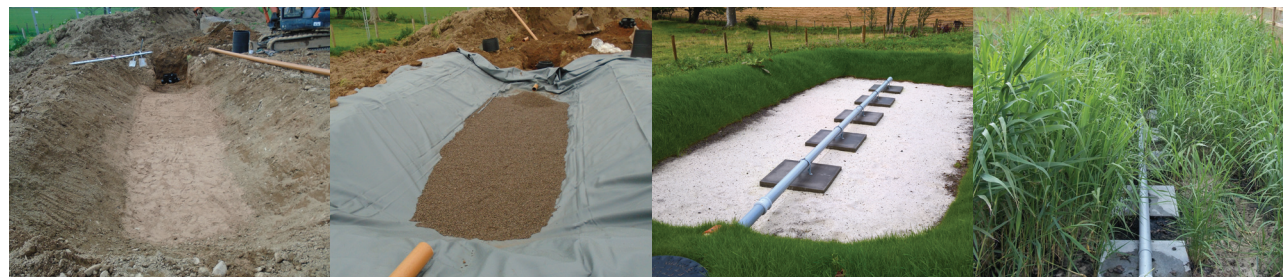
Sequence of activities in wetland construction. Photo courtesy of Moir Environmental
